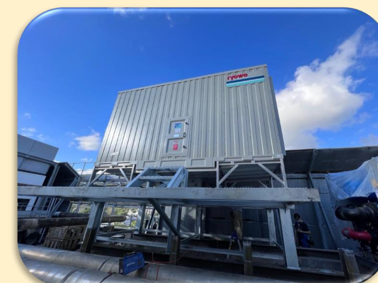
Figure 20: Conversion of Air-cooled Chiller to Water-cooled Chiller at EDB Kowloon Tong Education Services Centre in 2022
